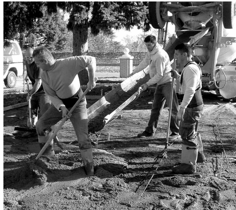
Pouring concrete for Omaha driveway
