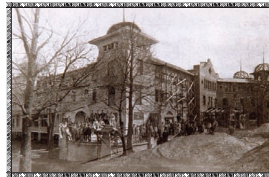
Construction of the "Hotel Colfax."
